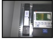
**2** - Using a flat Screw driver slide down the din-rail release clip and lift the bottom of the module away from the din-rail.
